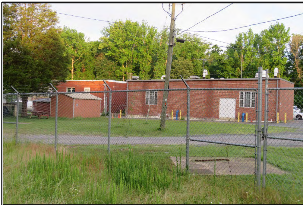
Figure 44. View of DHR #287-5004.
