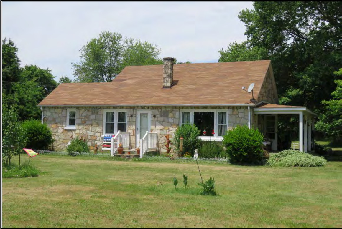
Figure 24. View of DHR #089-5333.
