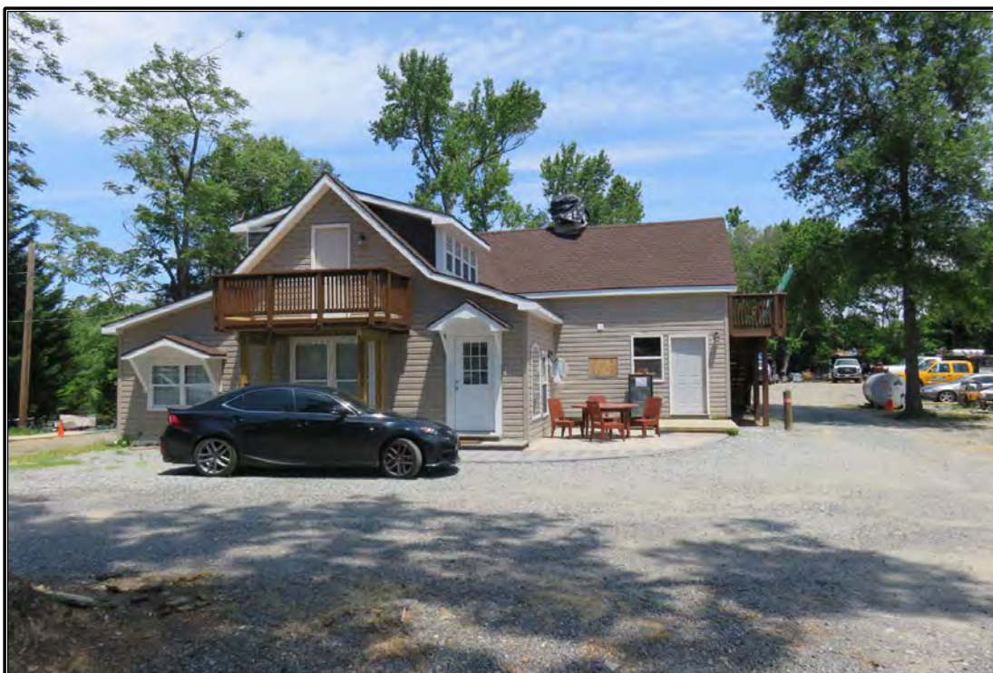
Figure 20. View of DHR #089-5295.
