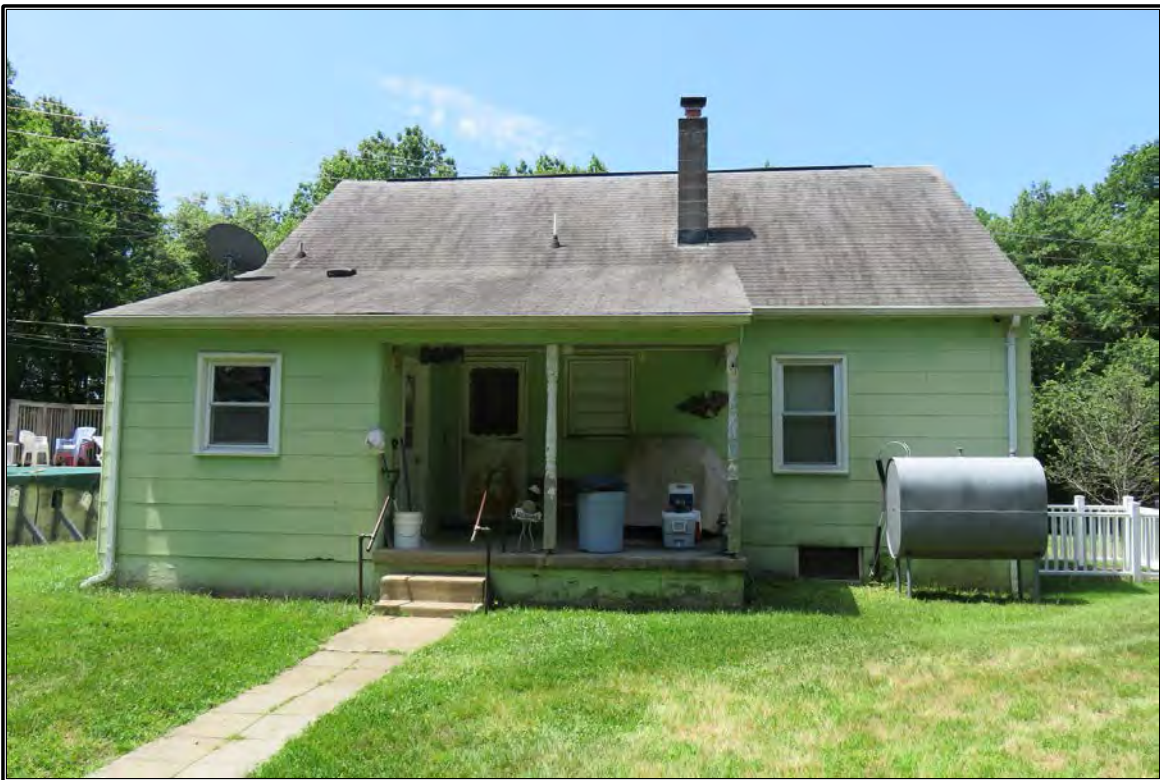
Figure 19. View of DHR #089-5294.
