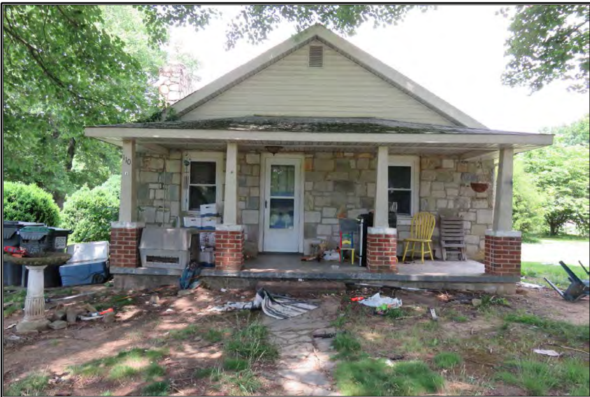
Figure 25. View of DHR #089-5334.
