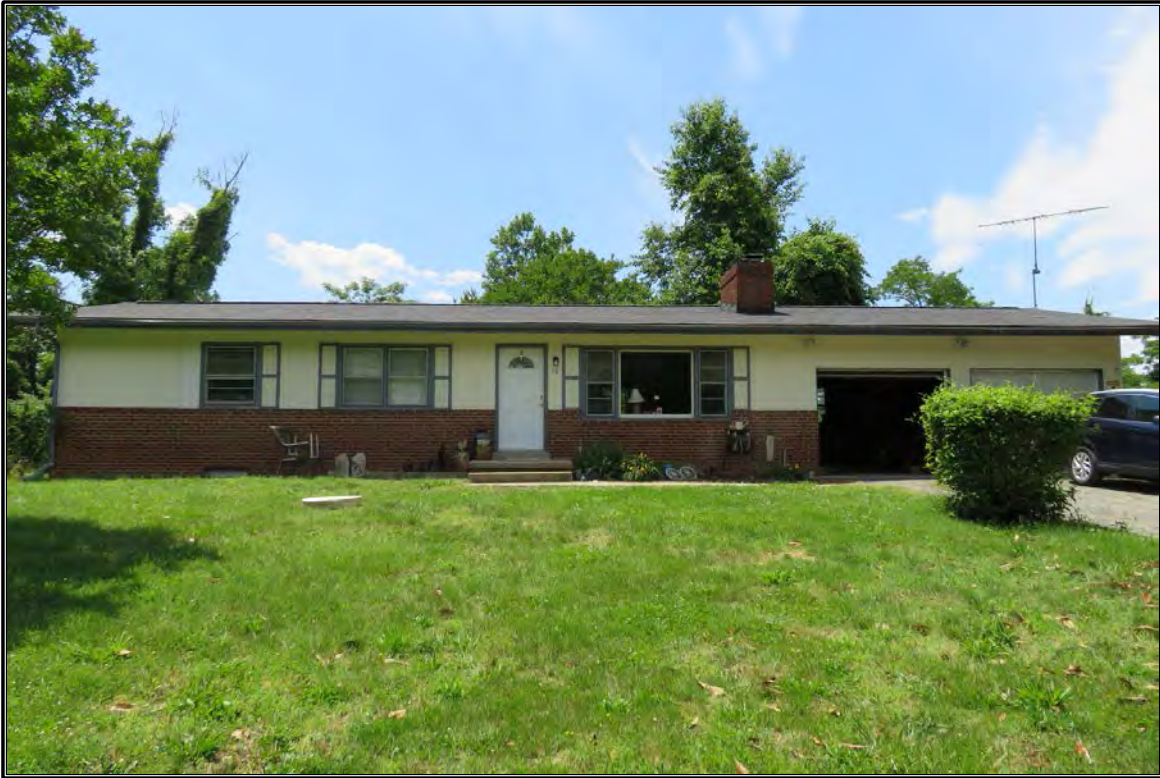
Figure 22. View of DHR #089-5331.
