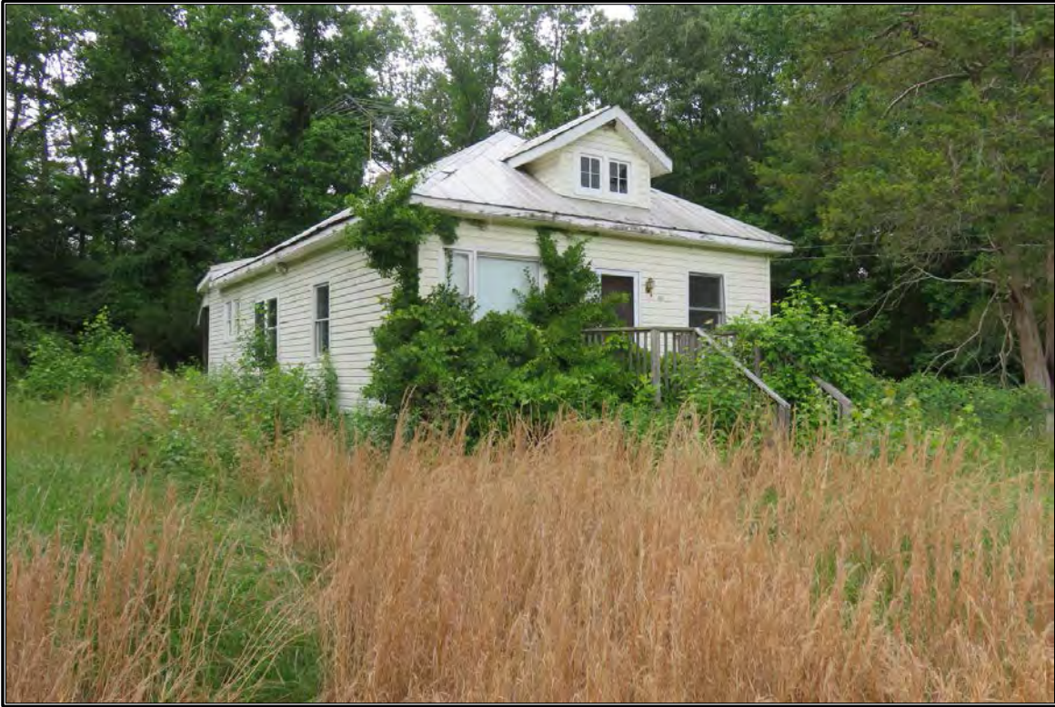
Figure 13. View of DHR #089-0327.
