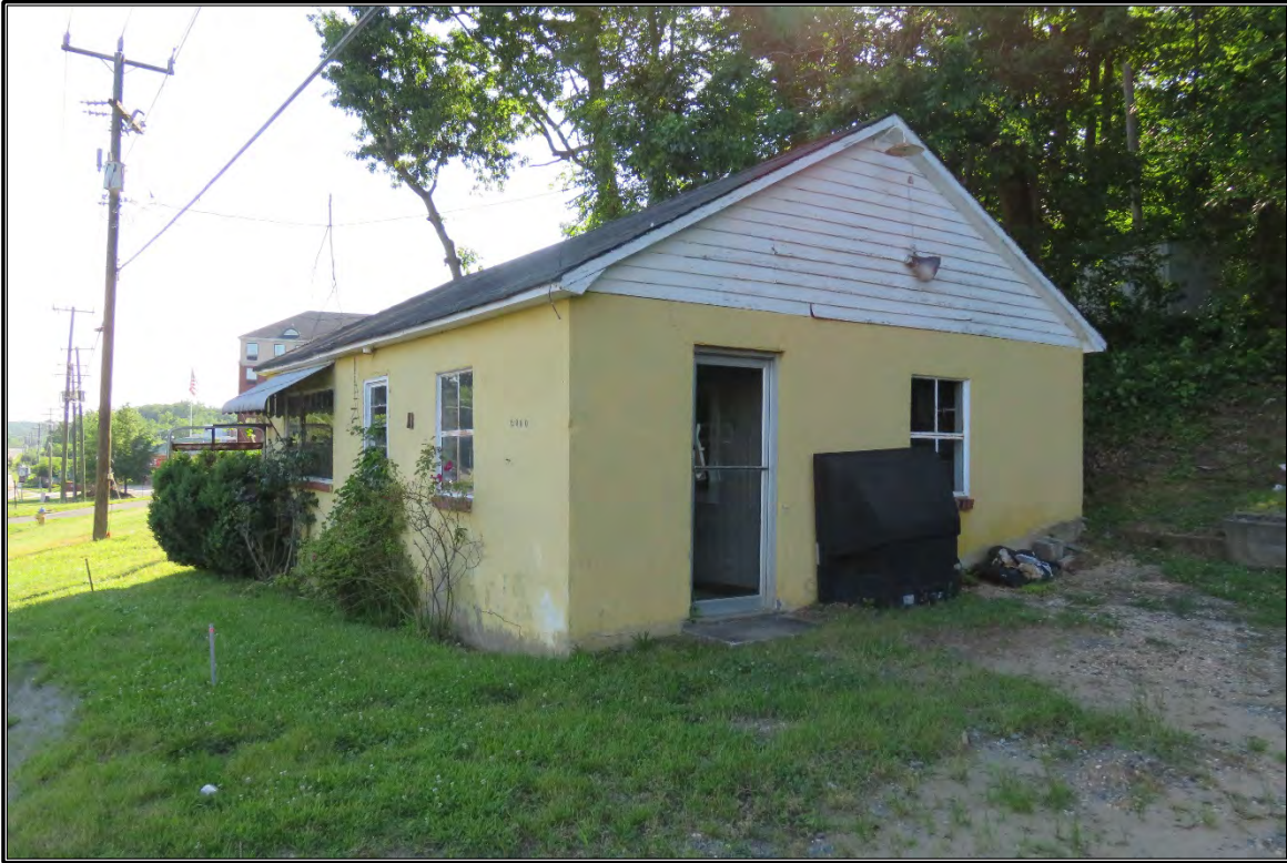
Figure 34. View of DHR #089-5612.
