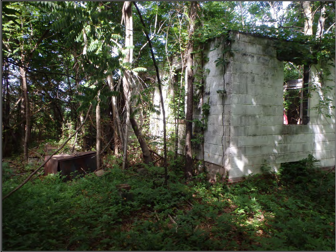
Figure 29. View of DHR # 089-5426.
