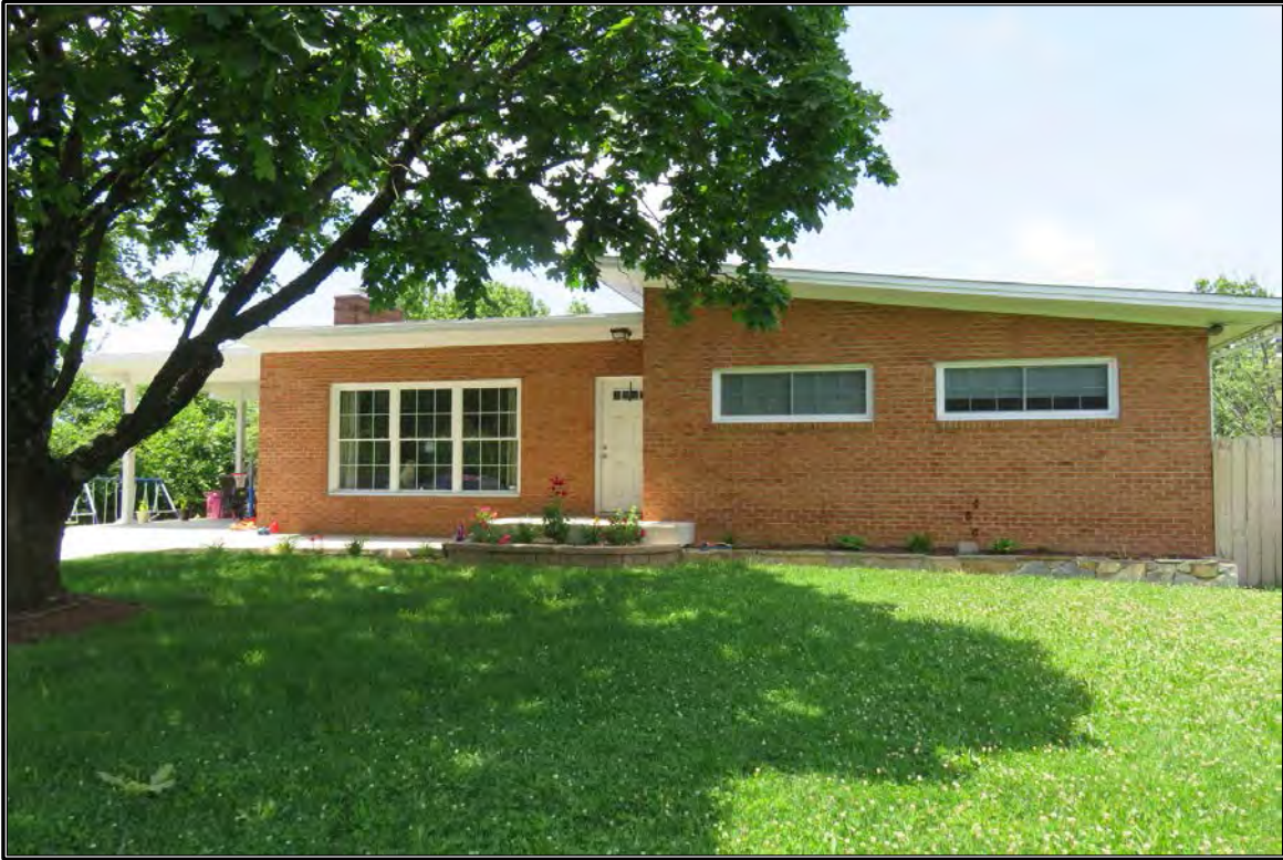
Figure 27. View of DHR #089-5373.
