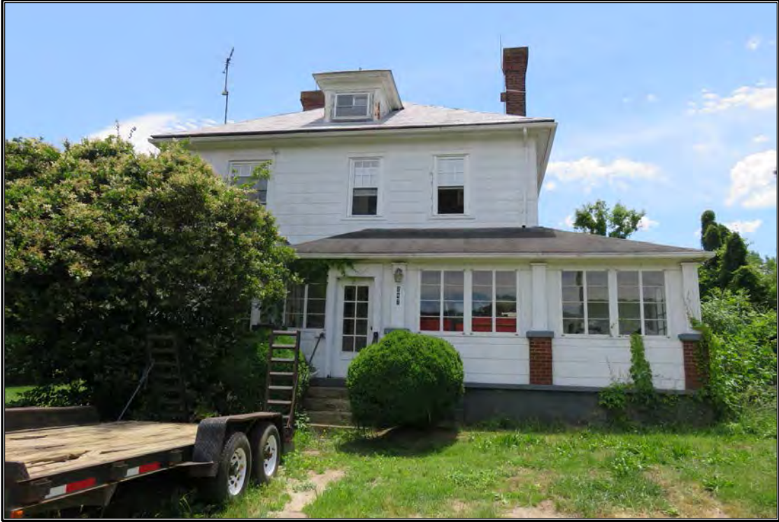
Figure 16. View of DHR #089-0364.
