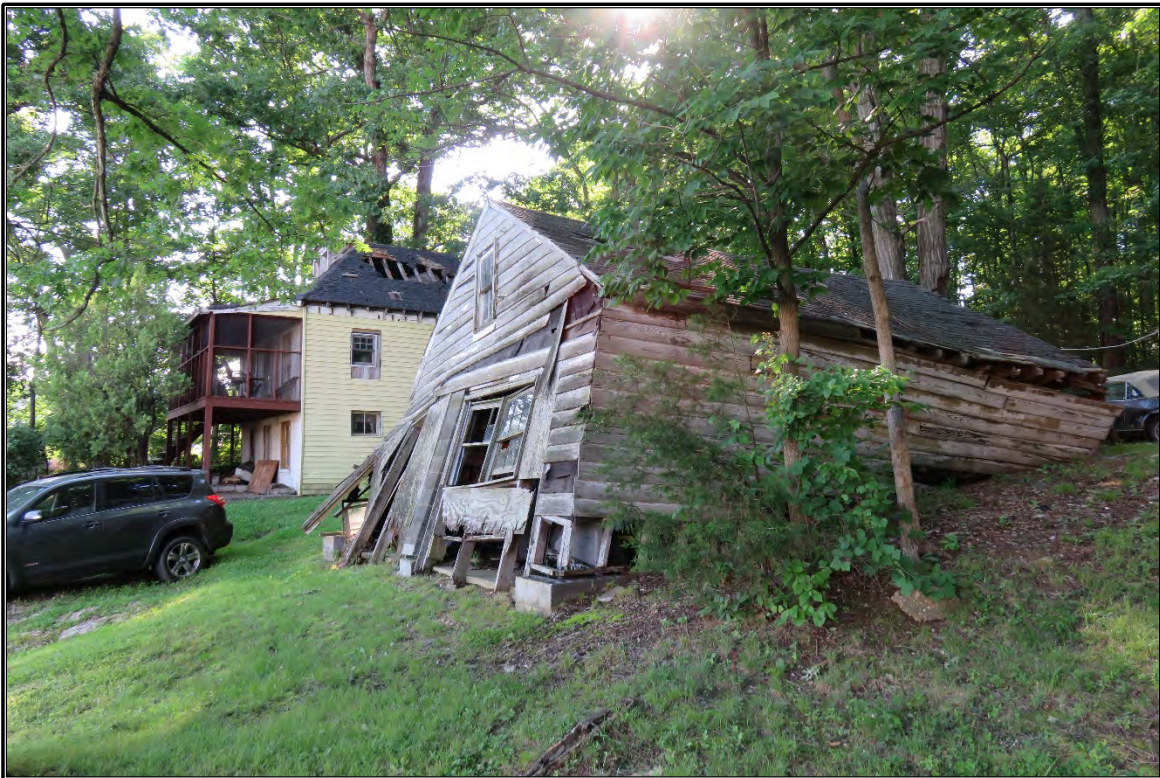
Figure 35. View of DHR #089-5613.
