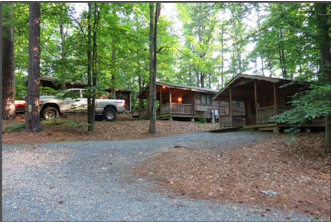
Figure 32. View of cabins associated with DHR #089-5610.
