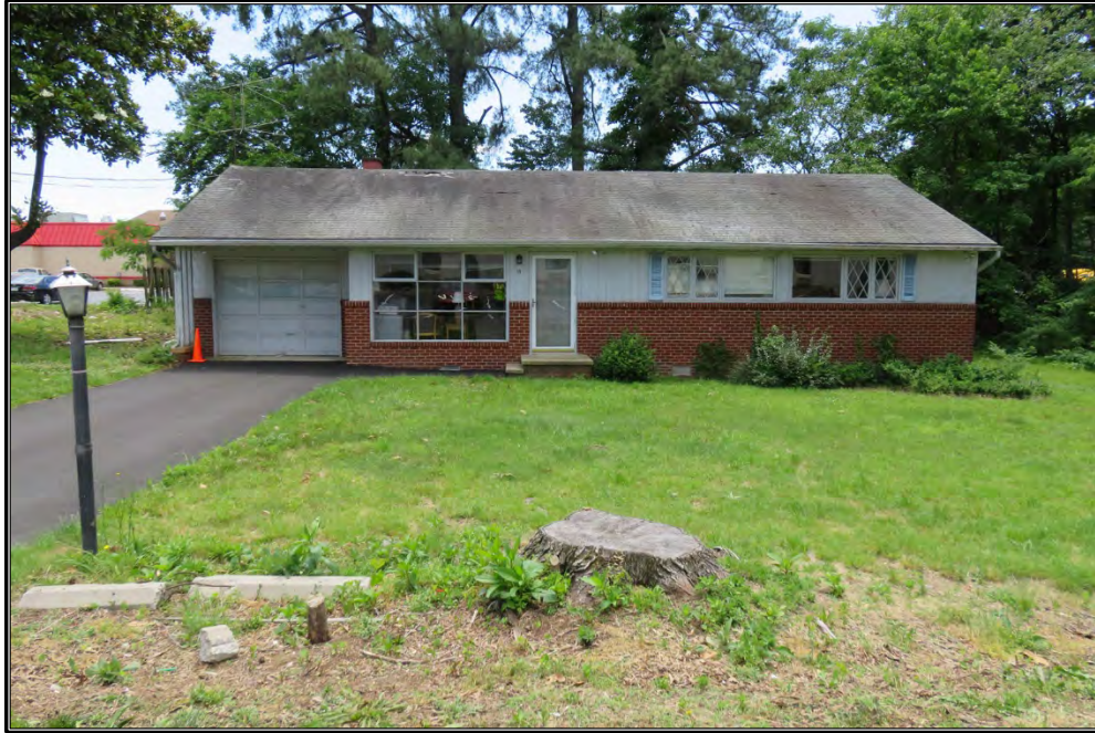
Figure 40. View of DHR #089-5618.
