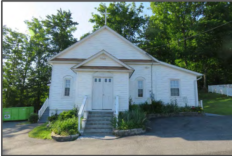
Figure 33. View of DHR #089-5611.
