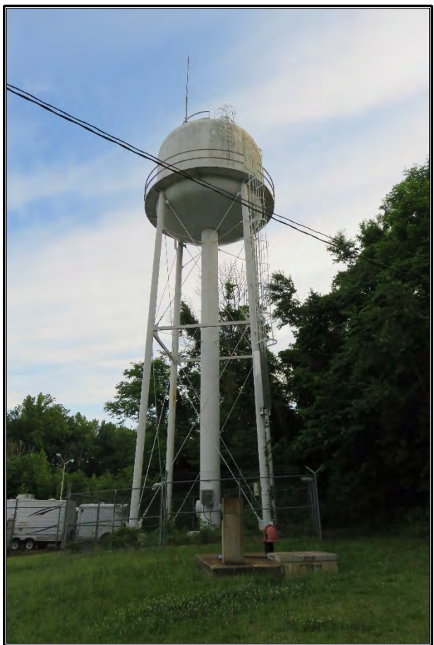
Figure 45. View of DHR #287-5148.
