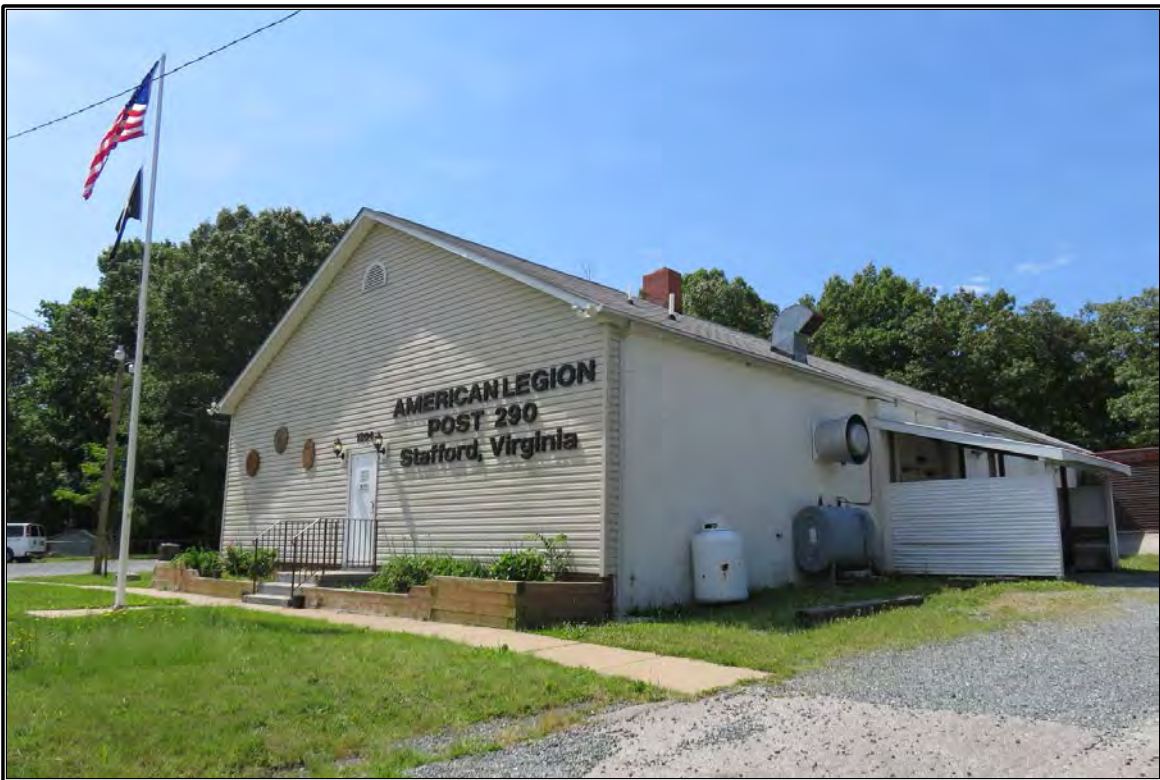
Figure 38. View of DHR #089-5616.
