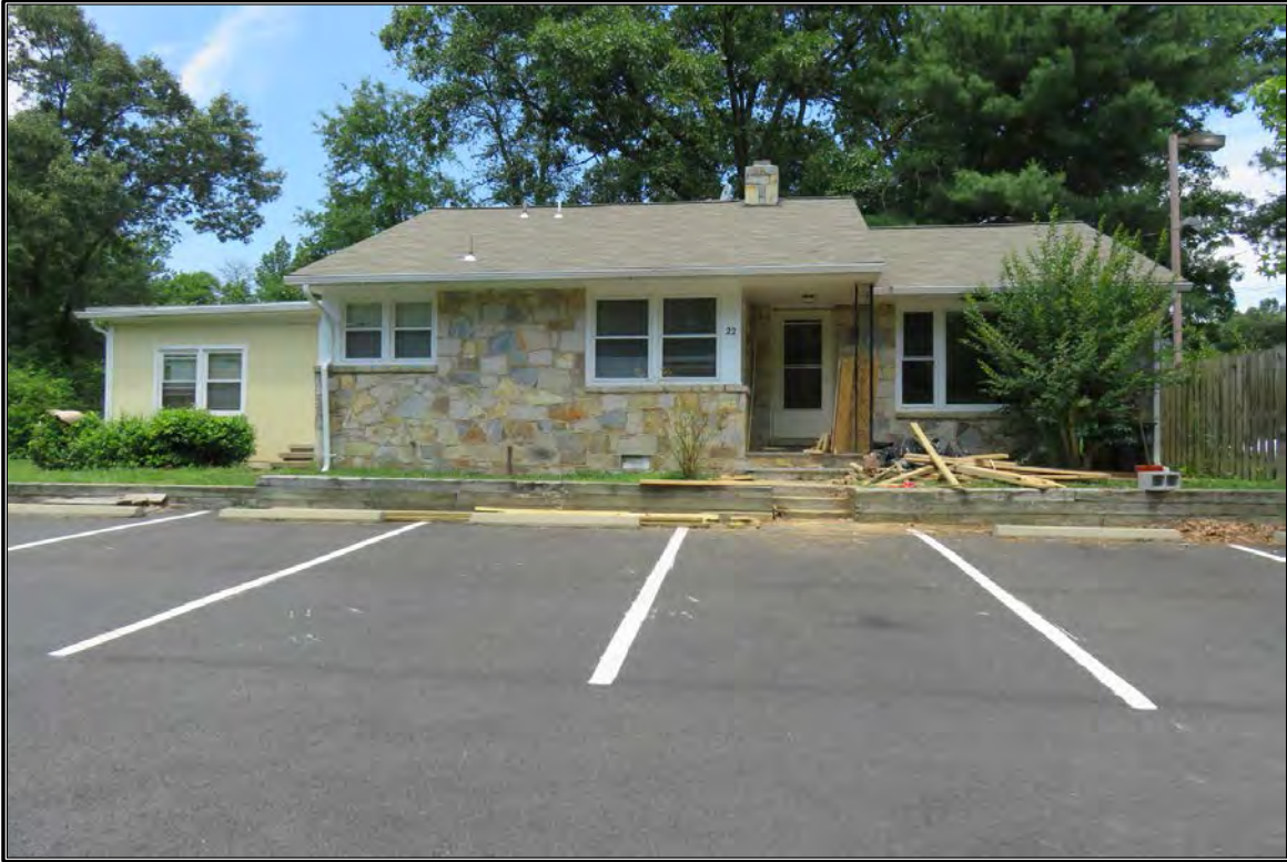
Figure 41. View of DHR #089-5619.
