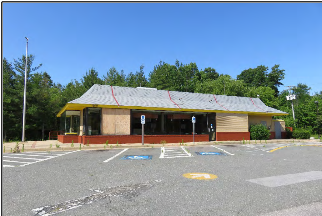
Figure 36. View of DHR #089-5614.
