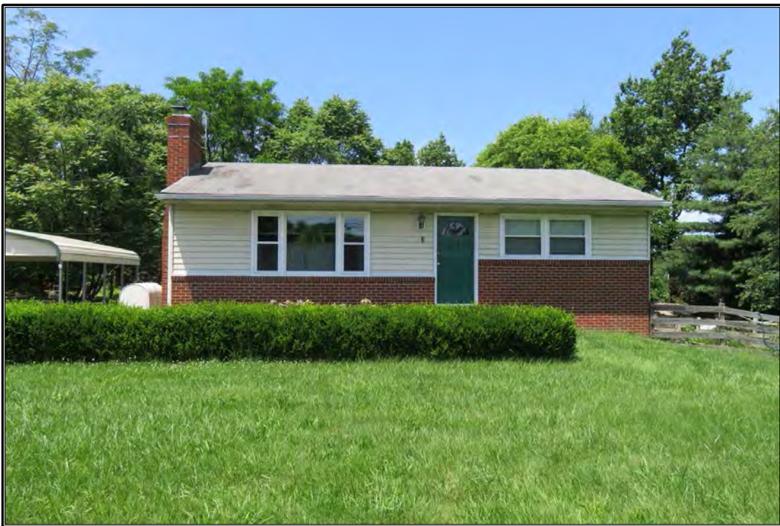
Figure 39. View of DHR #089-5617.
