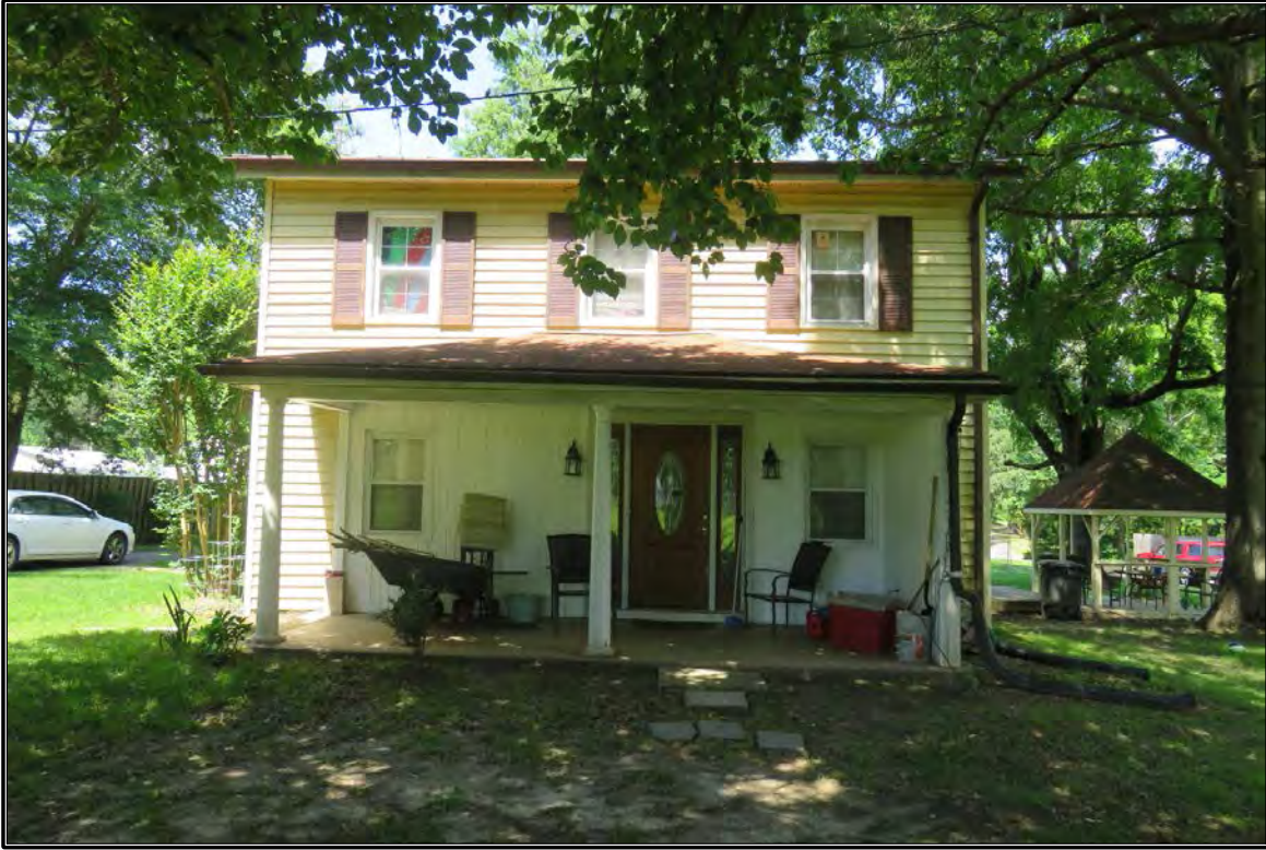
Figure 15. View of DHR #089-0330.
