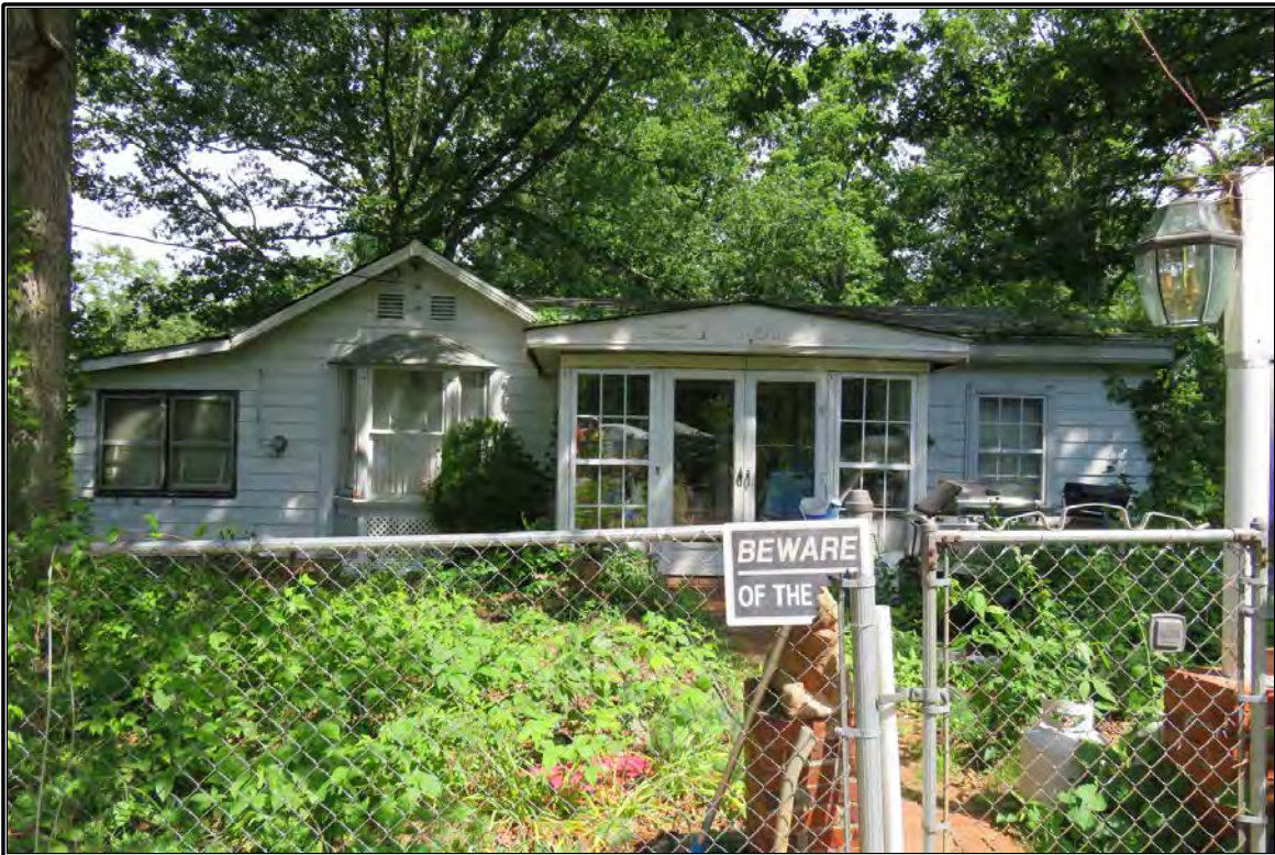
Figure 12. View of DHR #089-0325.
