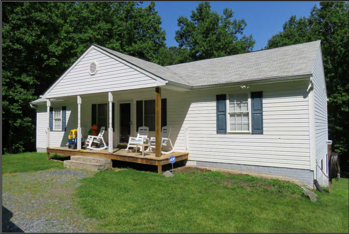
Figure 11. View of DHR #089-0324.
