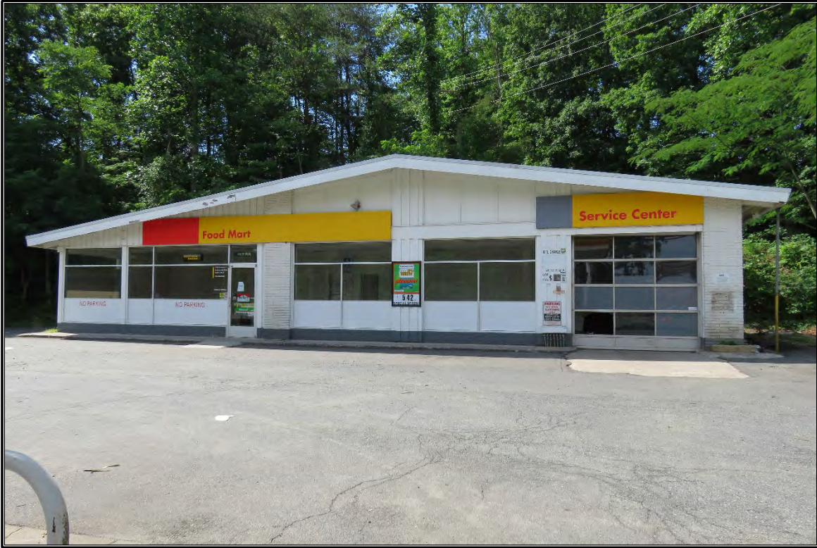
Figure 37. View of DHR #089-5615.
